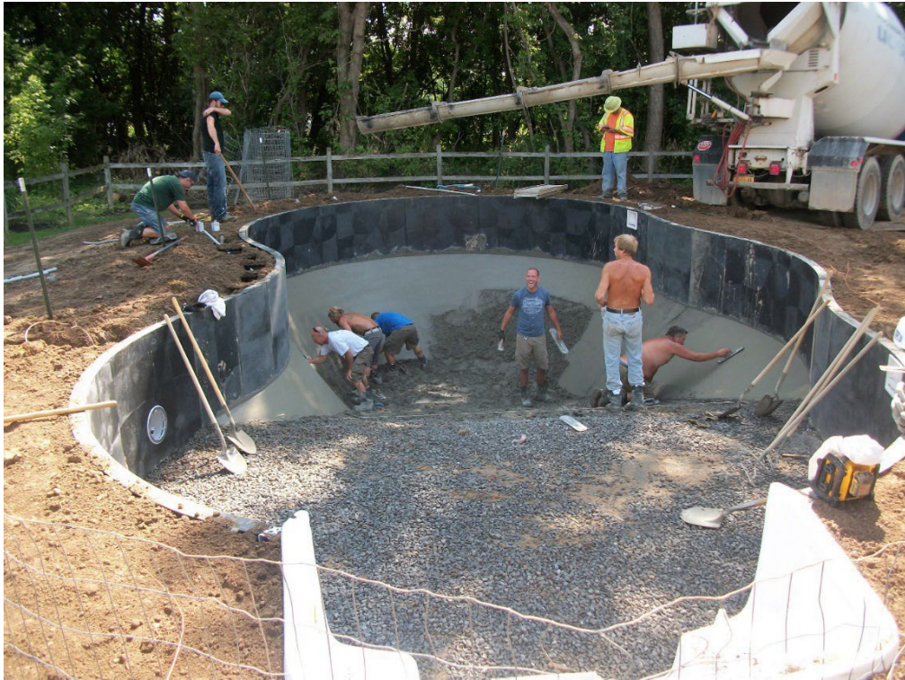
In this case, we put the bottom in after “plumb and backfill”.
