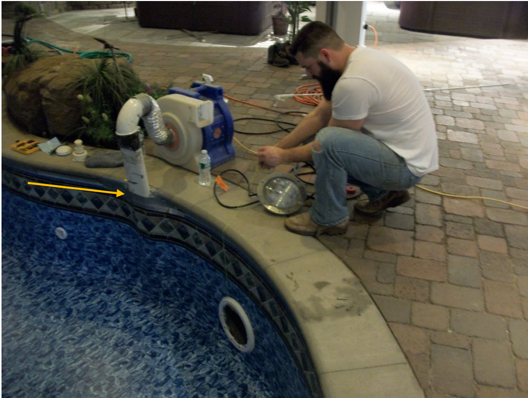
Here we are installing a new liner in one of our showroom pools. This pool has a 1' "bond beam" with a 3' subdeck. The pavers are installed over the top of the sub-deck. Note the "blower" and the tube behind the liner. The blower creates a strong vacuum to hold the liner in place while it is being filled.
