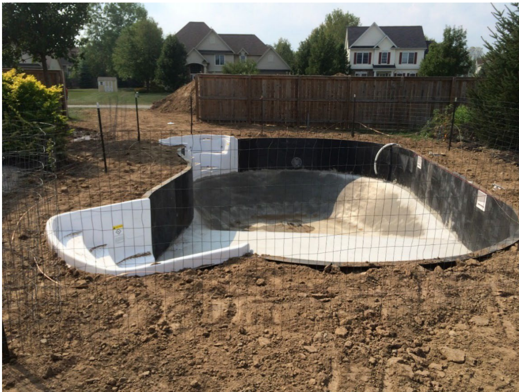
Generally, your yard will go from how it was to a structure, backfilled, plumbed and rough graded within one week. once it is backfilled, we will set up a temporary fence and you will be asked to set up “soaker hoses” to help settle the ground up near the pool.
