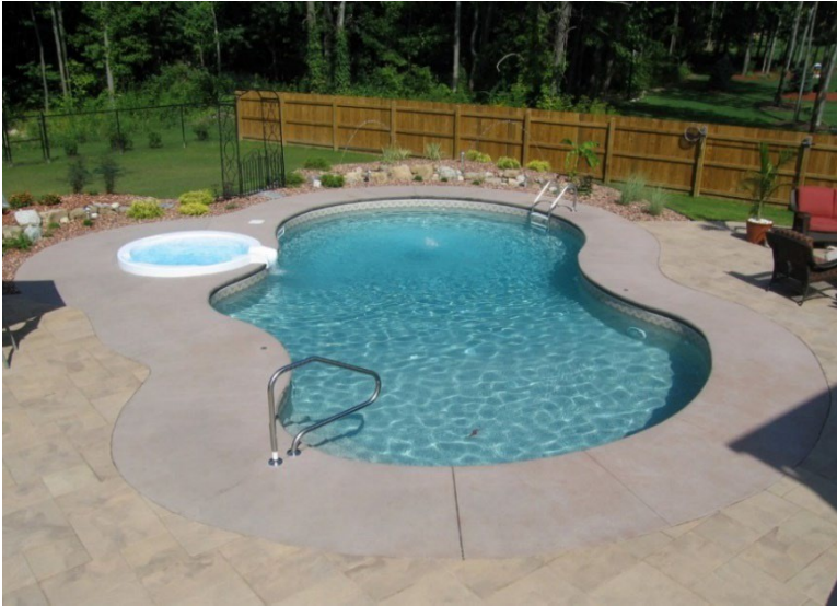
Here is a good example of pavers up to a colored concrete cantilever deck.
