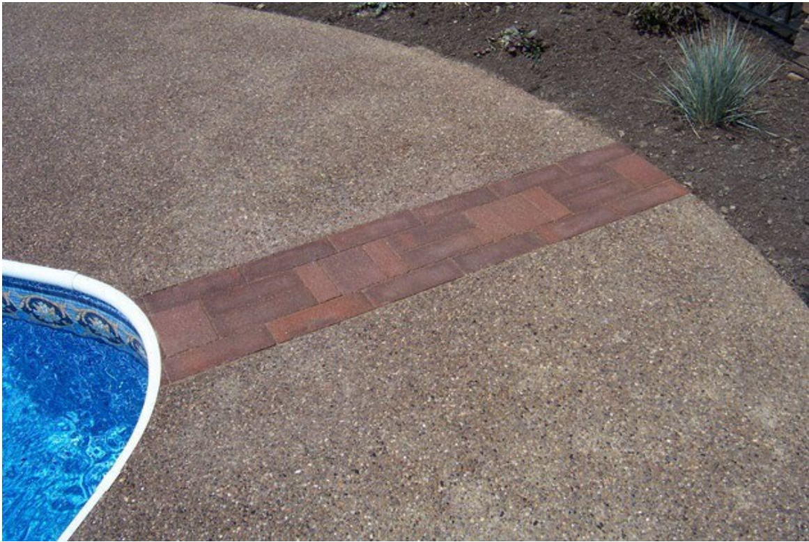
Here is an example of exposed aggregate with a brick design combo
