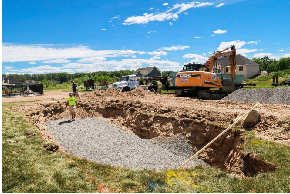
In this image, you can see that the site has been excavated and the crew is preparing to set the fiberglass pool.
