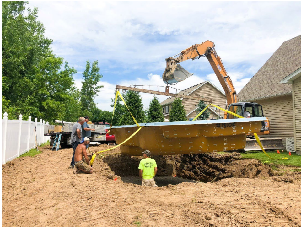
Here you can see that the crew is setting the fiberglass pool in the ground.
