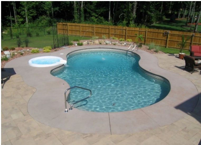
Here is a good example of pavers up to a colored concrete cantilever deck.
